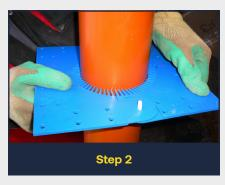
2 - Secure together with bolt and wing nut
