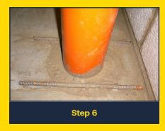
6 - Fill area with concrete and remove bars when set
