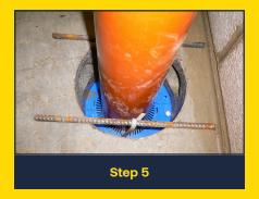
5 - Pull up the cable ties and secure into place
